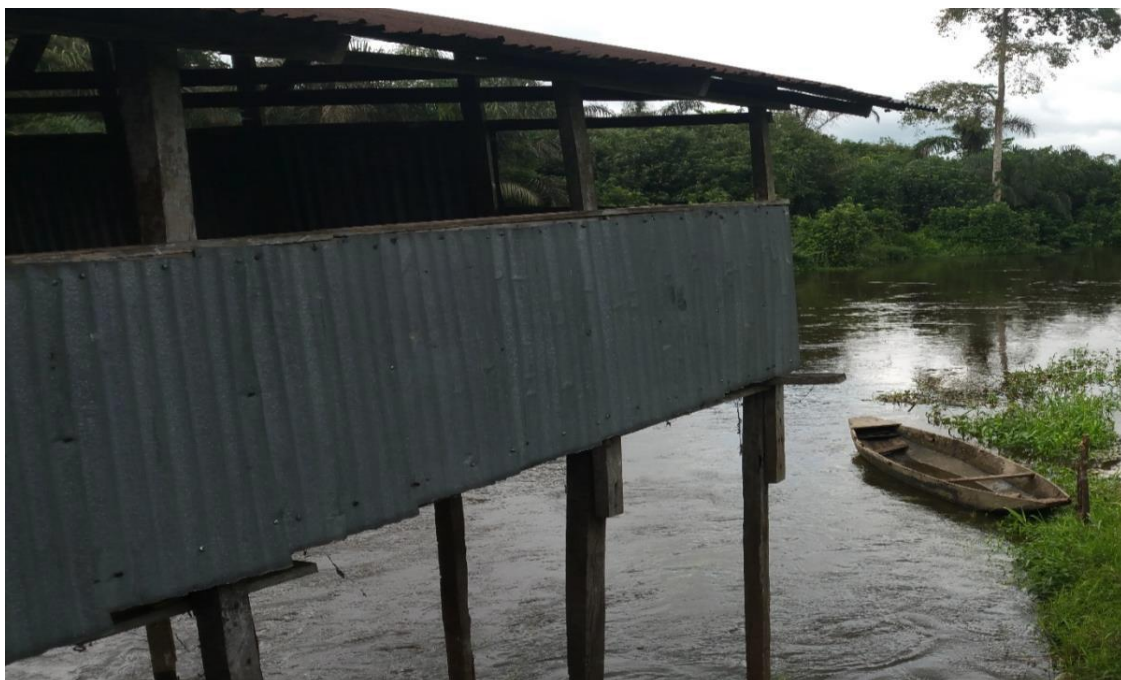
Figure 1c: Community Toilet Building Inside the River Overlooking the Sombrero River Channel.
