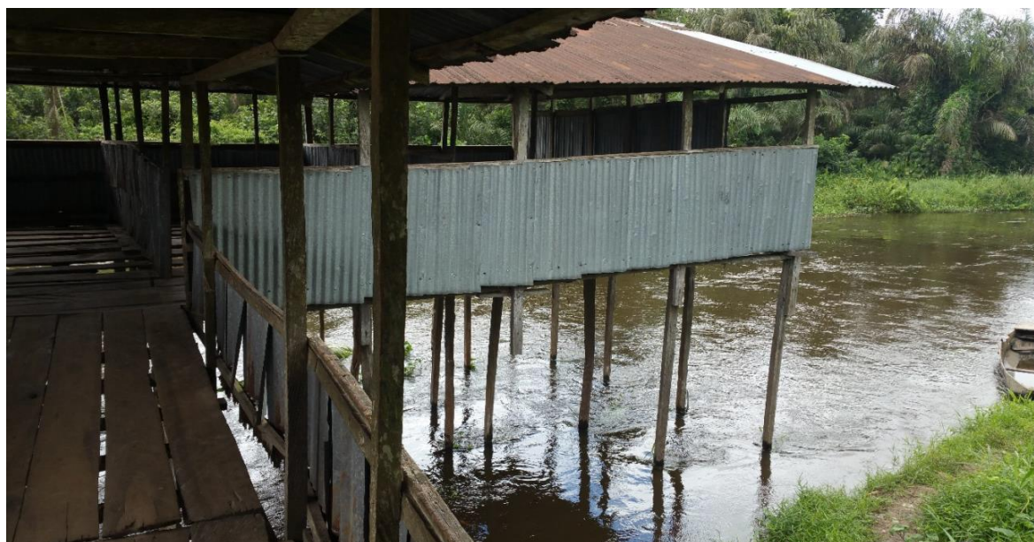
Figure 1e: Walkway to the Community Toilet inside the River.
