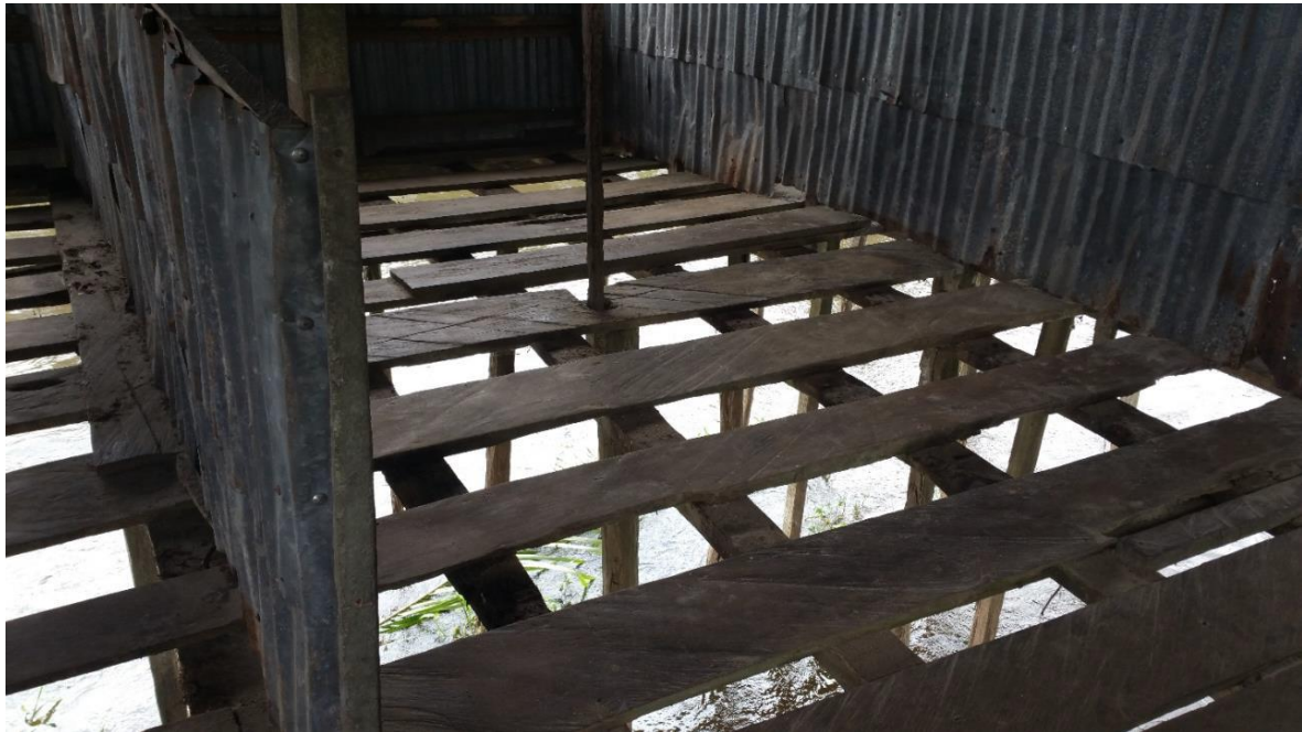
Figure 1d: Floor Wooden Platform of the Community Toilet in the Sombrero River Showing Openings for Faeces Droppings into the River Beneath.
