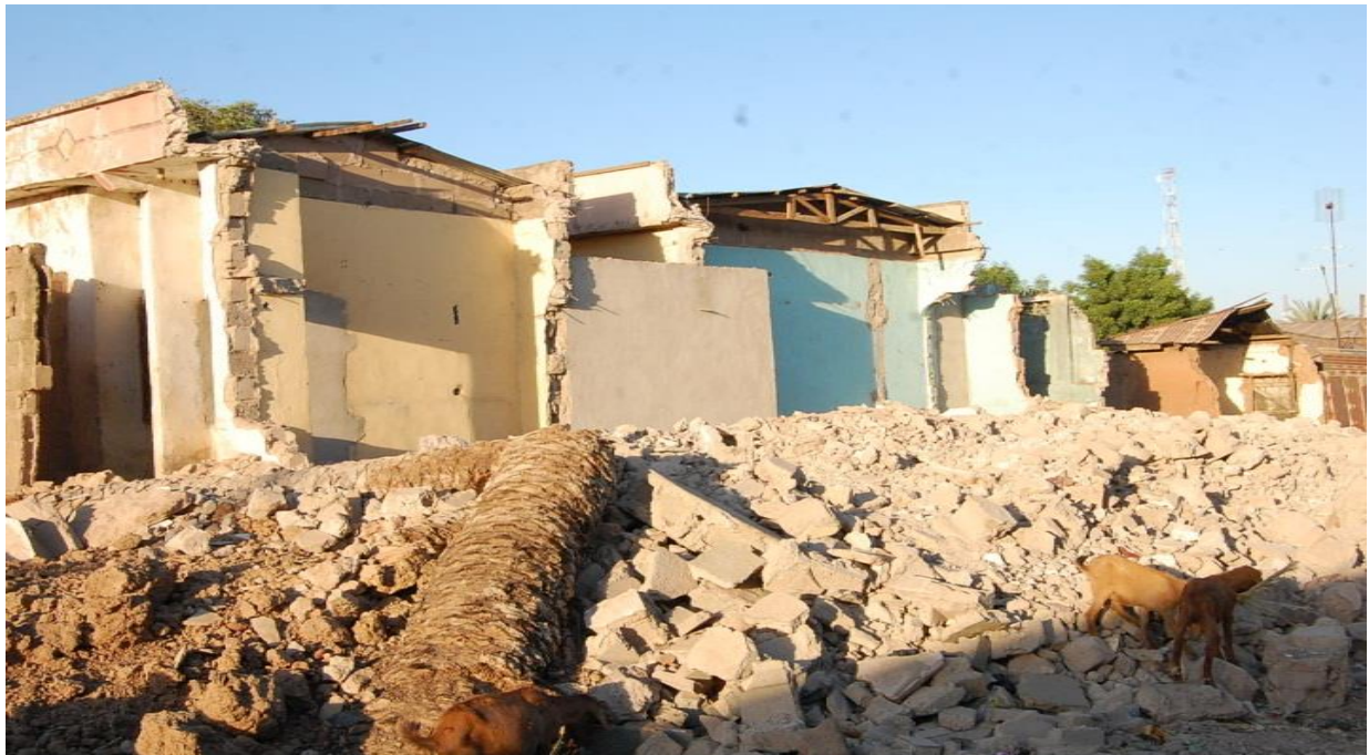
Plate 2: Sandcrete based demolition debris on Idi road 6 in Lot 1
