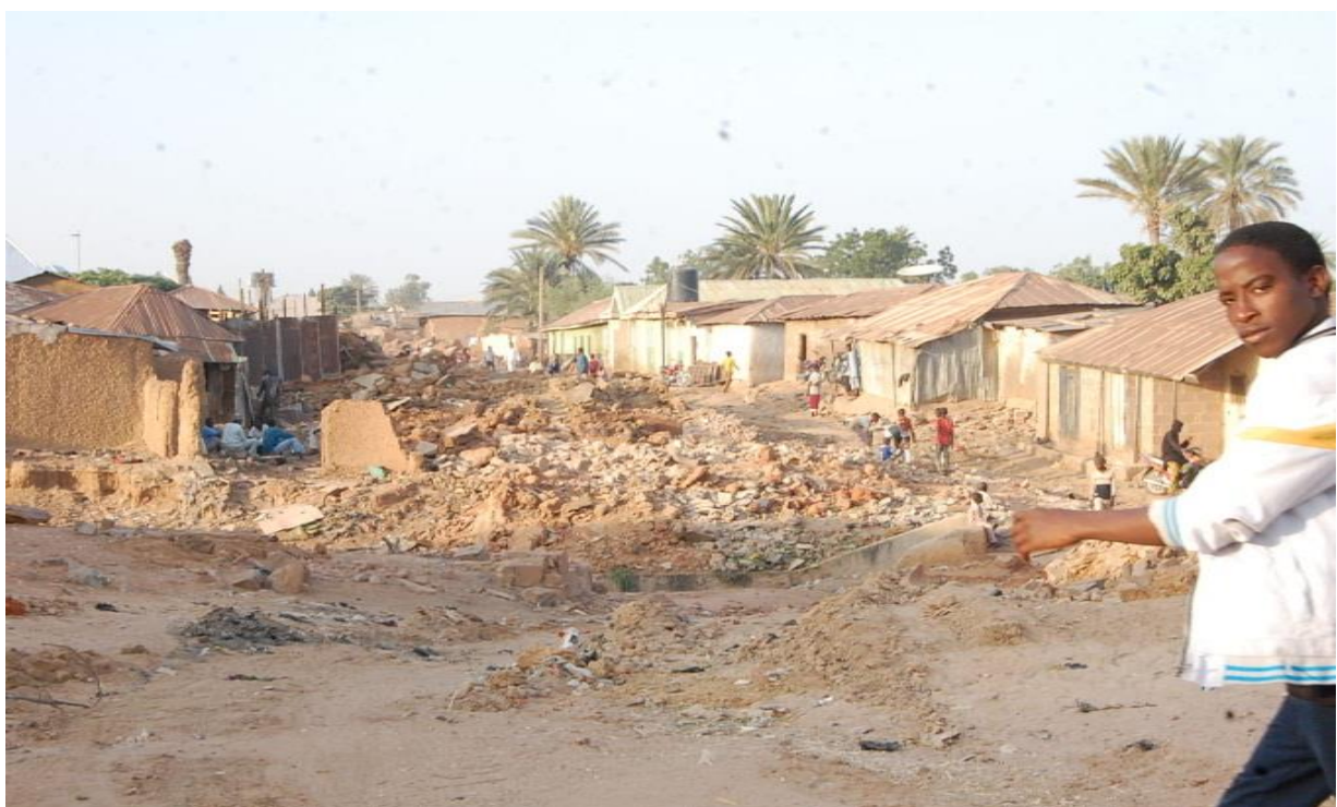
Plate 3: Clay based material from demolition on liberty-G/hospital road 1 in Lot 1
