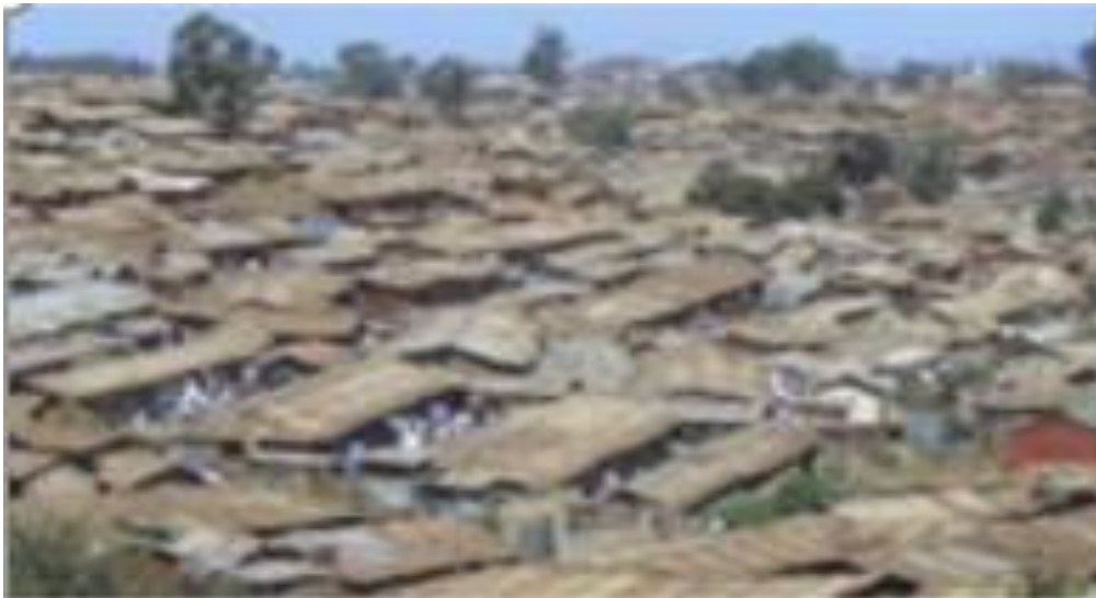
Figure 7: Crowded Slum Settlement Arise from Absence of Effective Special Planning and Development Control Source: Field Study in Abuja FCT, 2019
