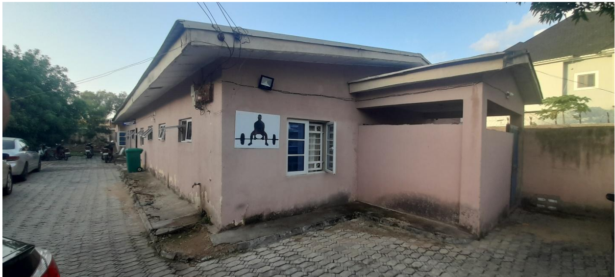
Plate 2: 02 fitness and physiotherapy center Bauchi is poorly lighted and ventilated.
