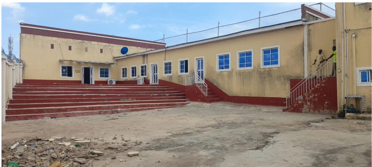
Plate 3: Babayo Liman Sport Arena; Bauchi is poorly lighted and ventilated
