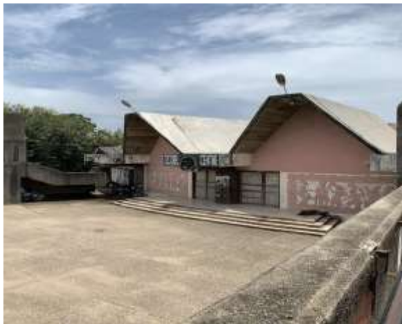
Figure 8. Interior courtyard of the Cultural Centre, Mokola (Photograph by Author, 2025).
