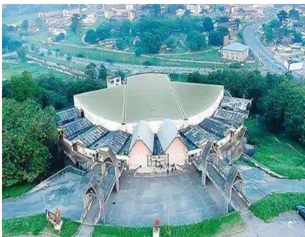
Figure 6. Exterior view of the Cultural Centre, Mokola (Photograph by Author, 2025).
