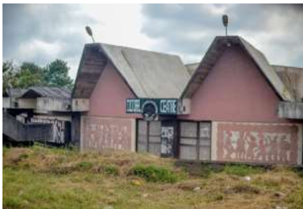
Figure 1. Front view of the Cultural Centre, Mokola, Ibadan (Photograph by Author, 2025).
