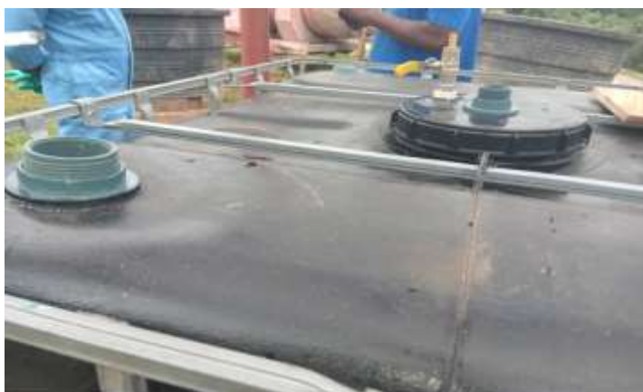
Figure 8: Pipe Assembly into the cut holes
