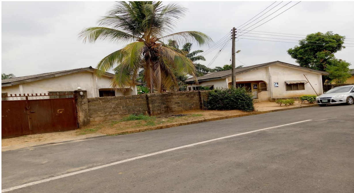
Plate 5: The Detached 3 - bedroom bungalow at AHOCOL Oganiru Housing Estate, Agu-Awka (AHOCOL 3) showing its appearance as a full-provision house rather than a partial-provision type (core house).
