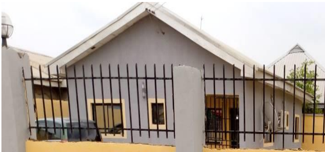
Plate 7: Detached 1- bedroom bungalow (Core House) at ASHDC Ngozika Housing Estate, Phase 1, Ikwodiaku, Awka (NGOZIKA 1) showing its appearance as a full-provision house rather than a partial-provision type (core house).
