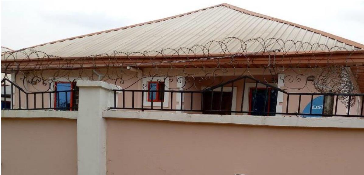
Plate 8: Detached 2- bedroom bungalow (Core House) at ASHDC Ngozika Housing Estate, Phase 1, Ikwodiaku, Awka (NGOZIKA 1) showing its appearance as a full-provision house rather than a partial-provision type (core house).
