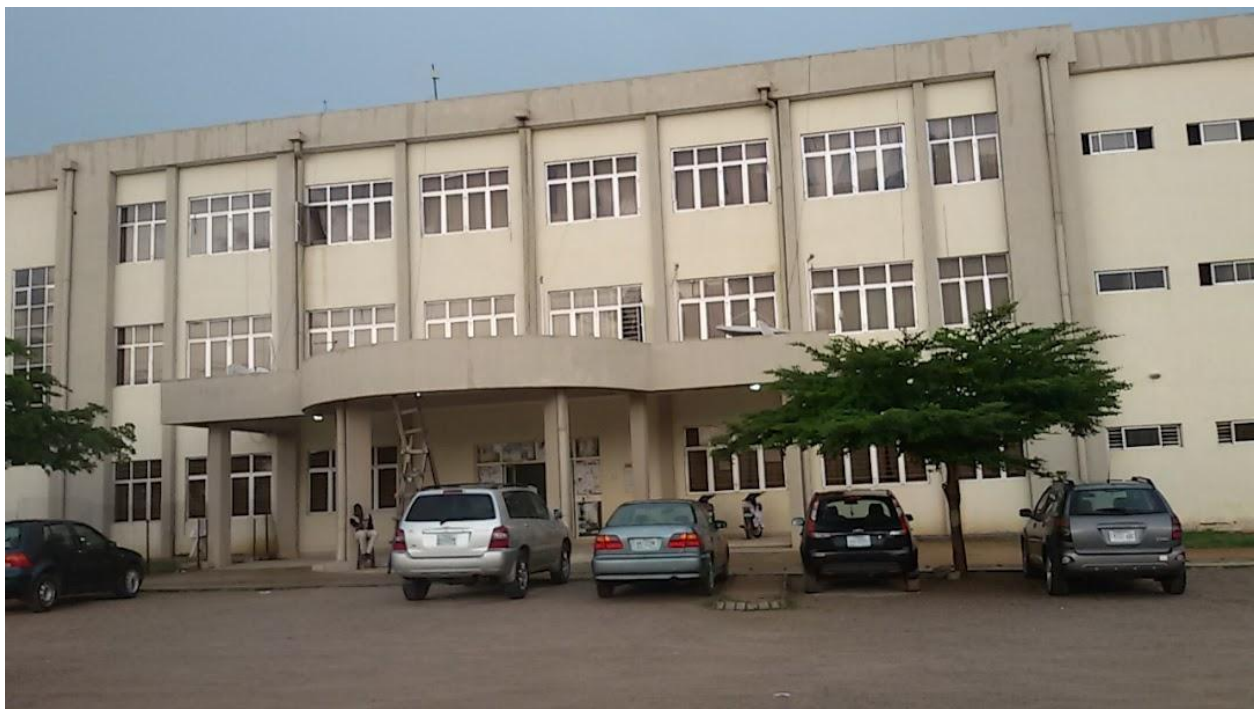
Figure 1: Faculty of Environmental Technology, Phase II
