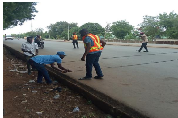
Figure 3: Installation of Pneumatic tubes
