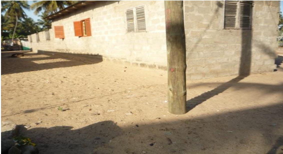
Fig 3.3 CCA treated poles sited around residential facilities
