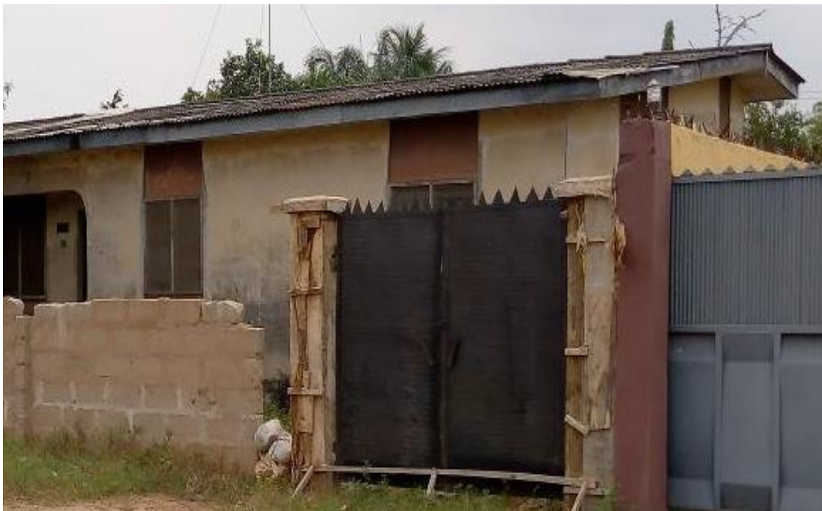
Plate 2: Photographic Image of the Semi-detached 3-Bedroom Bungalow at AHOCOL Phase 2 (AHOCOL 2) showing Cement Block Wall Material and Corrugated Asbestos Sheets as Roof Covering.
