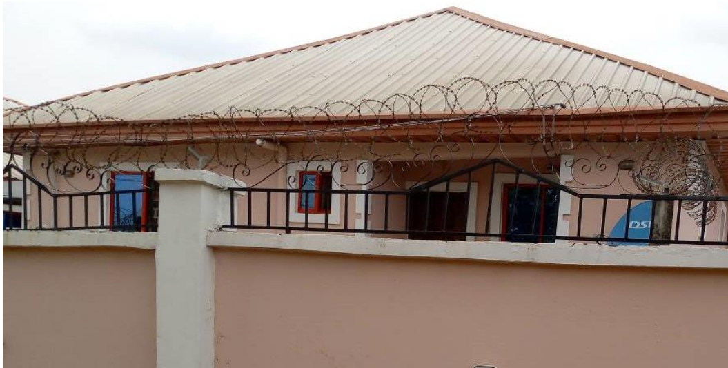
Plate 8: Detached 2- bedroom bungalow (Core House) at ASHDC Ngozika Housing Estate, Phase 1, Ikwodiaku, Awka (NGOZIKA 1) showing its appearance as a full-provision house rather than a partial-provision type (core house).
