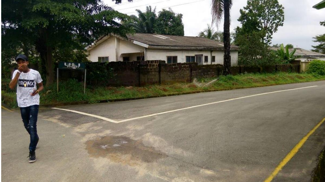
Plate 2: The Detached 3 - bedroom bungalow at AHOCOL Oganiru Housing Estate, Agu-Awka (AHOCOL 3) showing Cement Block Wall Material and Corrugated Asbestos Sheets as Roof Covering
