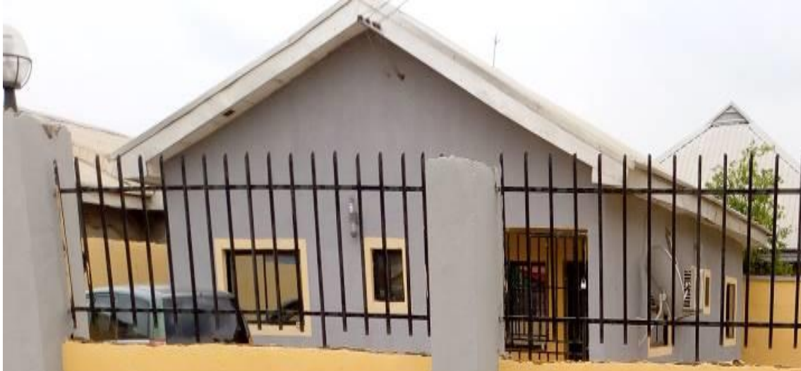
Plate 7: Detached 1- bedroom bungalow (Core House) at ASHDC Ngozika Housing Estate, Phase 1, Ikwodiaku, Awka (NGOZIKA 1) showing Cement Block Wall Material and Longspan Aluminum as Roof Covering.
