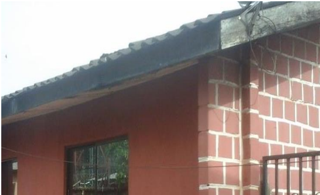
Plate 6: Detached 2- bedroom bungalow (Core House) at AHOCOL Inner City Layout, Nkwelle, Awka (AHOCOL 4) showing Cement Block Wall Material, Oven-baked brick for Front Wall and Clay tiles as Roof Covering
