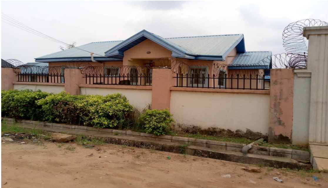
Plate 9: Detached 3 - bedroom bungalow (Core House) at ASHDC Ngozika Housing Estate, Phase 1, Ikwodiaku, Awka (NGOZIKA 3) showing Cement Block Wall Material and longspan aluminum as Roof Covering
